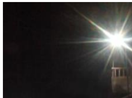
Solar lights are turned on automatically at night
