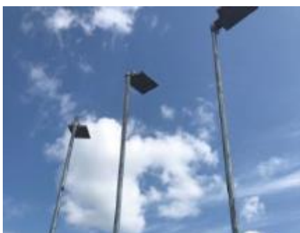
The installed solar lights
