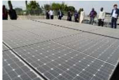
Inspection of Solar system At Usman Dam
