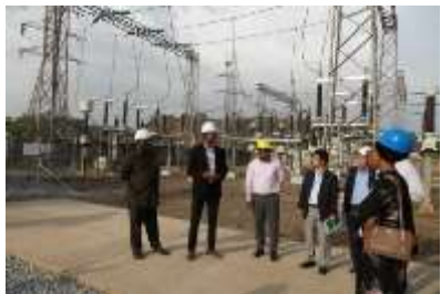
Inspection of Power system At Apo
