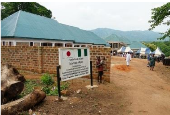
The newly constructed vocational training centre
