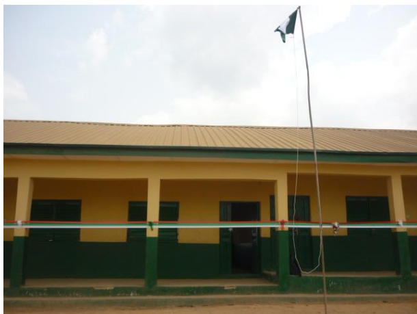
Newly constructed school block
