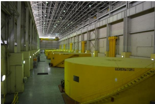
Inside of the Jebba Hydro Power Station
