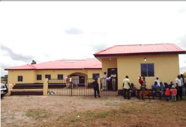
Newly Constructed Primary Health Centre
