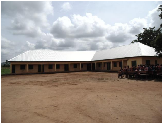
Newly constructed classrooms
