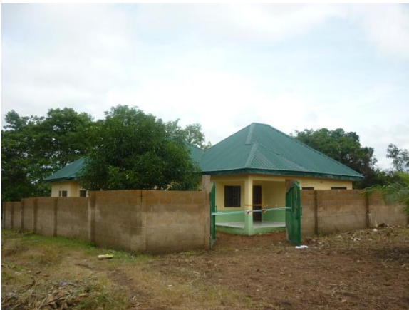
Newly constructed Health Clinic
